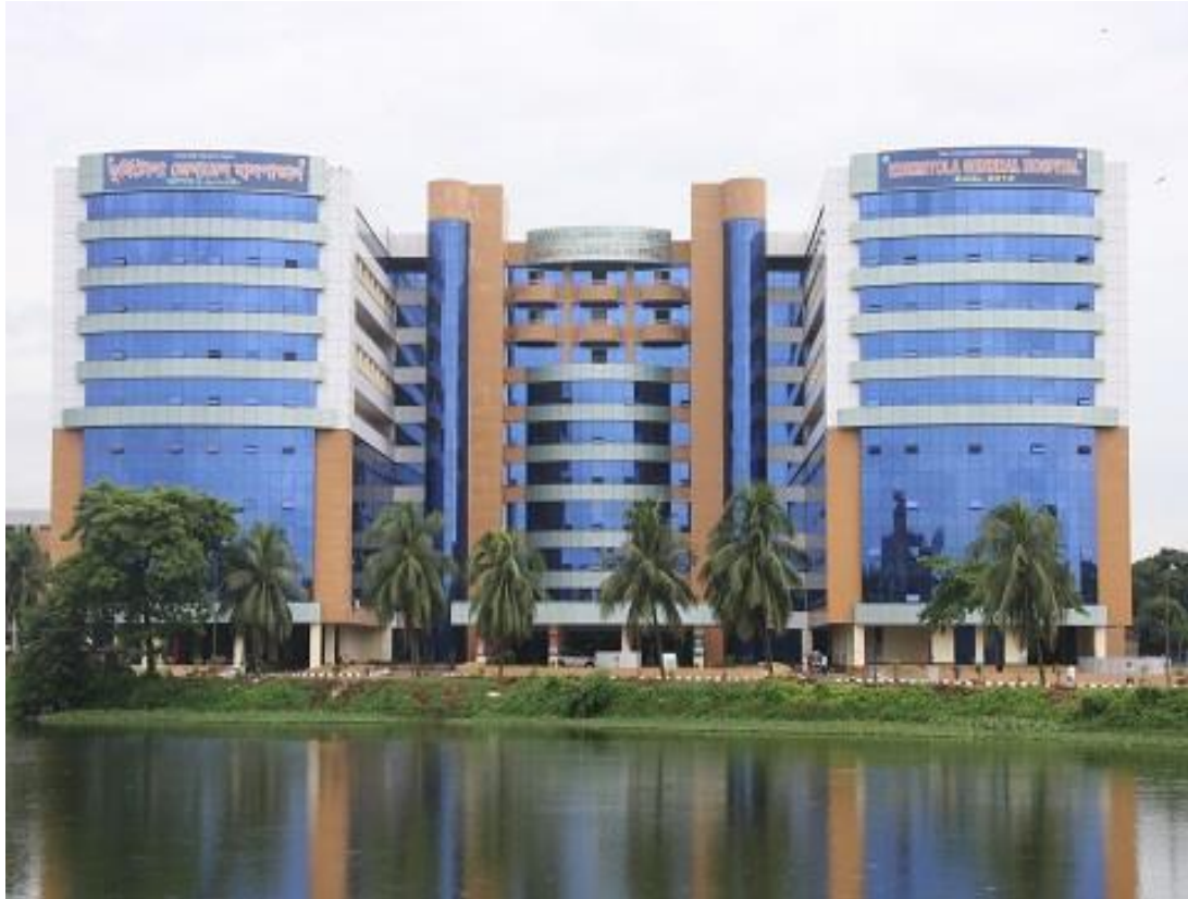
500 Bedded Kurmitola General Hospital Dhaka
