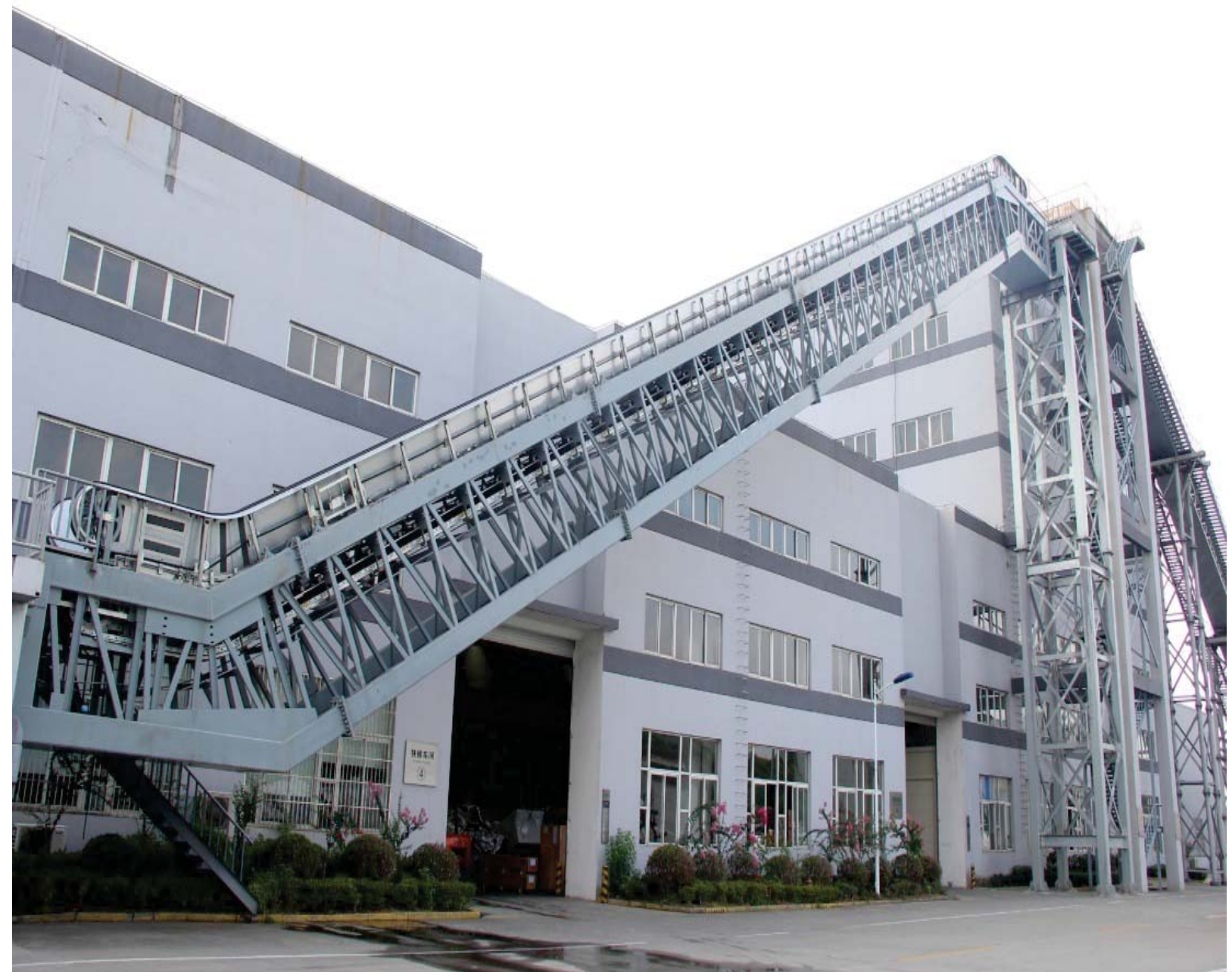
20 meters rise without intermediate support
