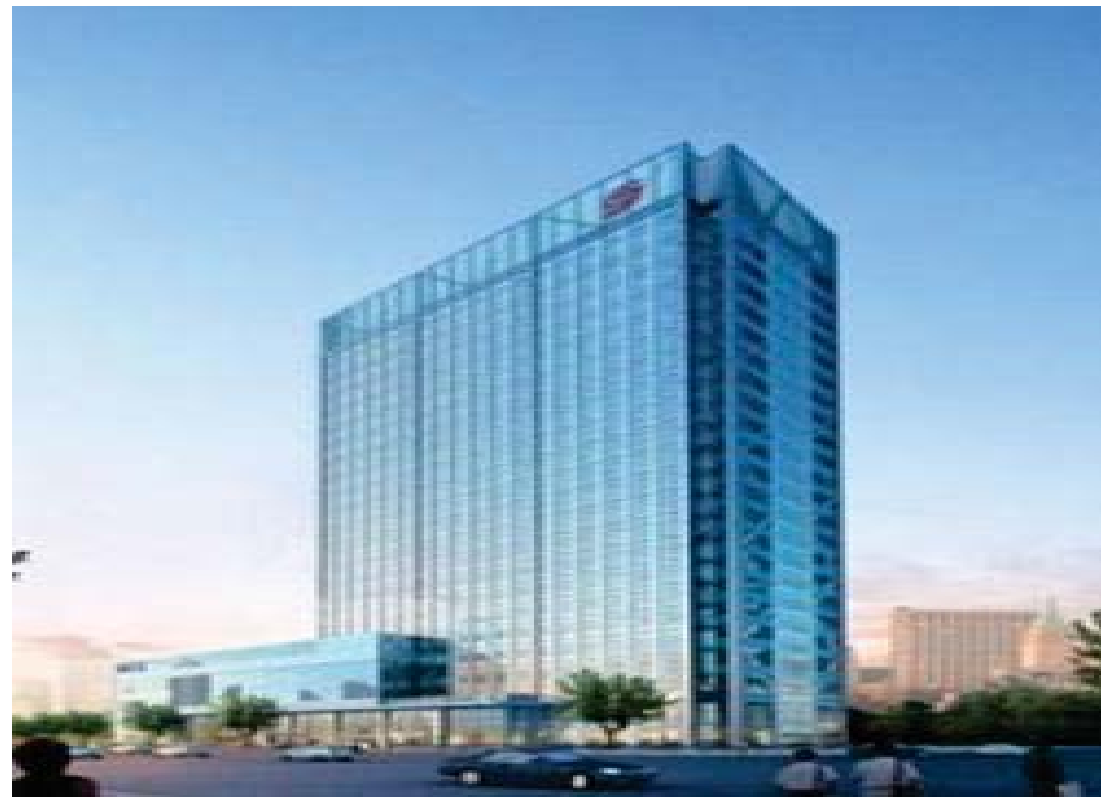
Suzhou Metro Control Center 3.5m/s
