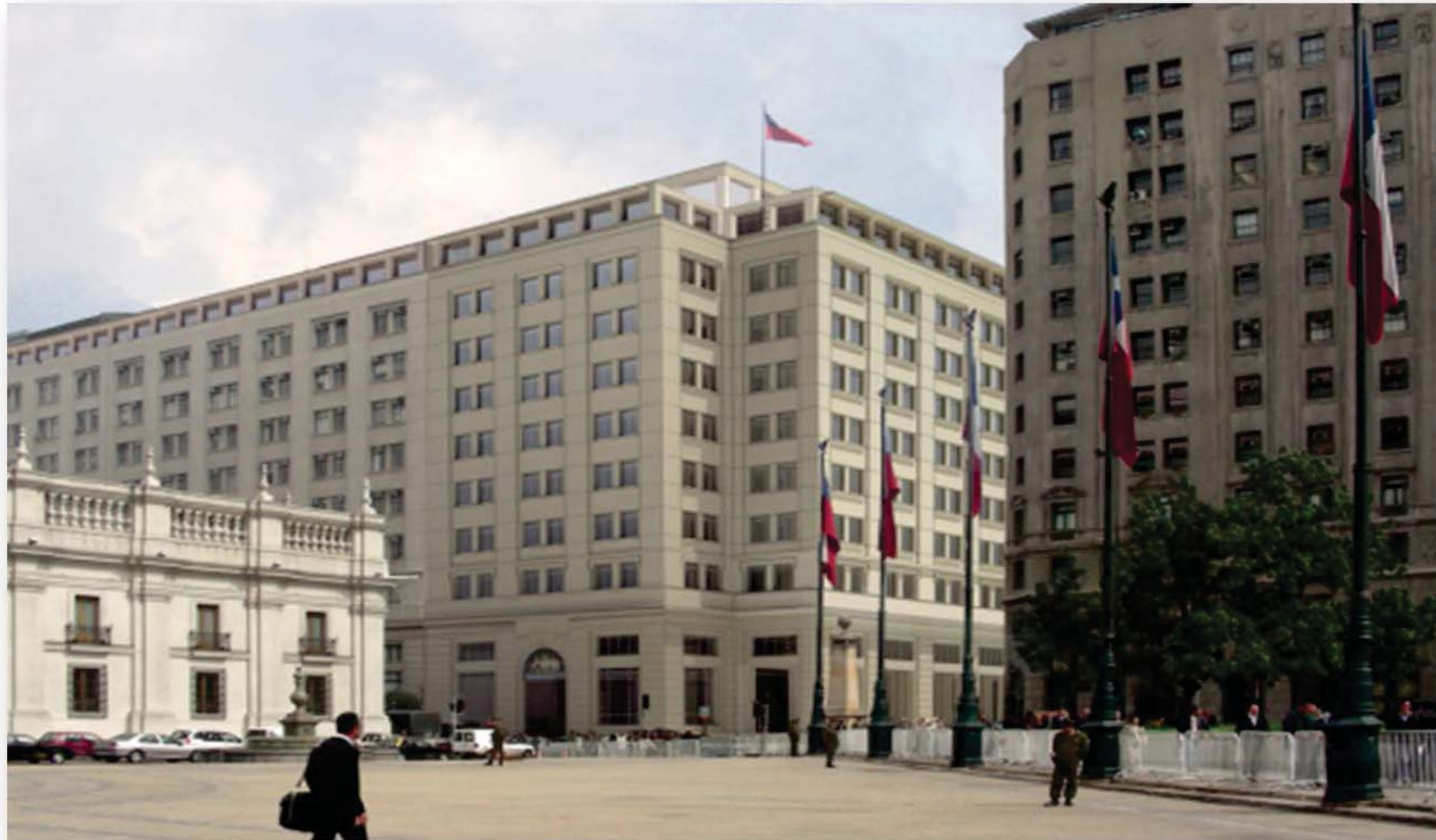
Chile Governmental Center Building
